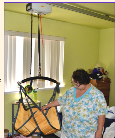
Marcia demonstrates use of the lift system, the track attached to the ceiling above her
